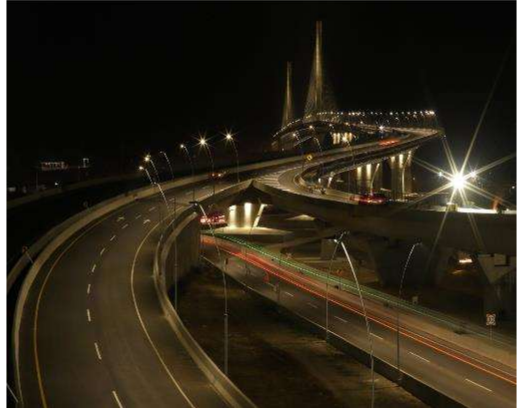
Pumarejo Bridge - Barranquilla - Colombia
